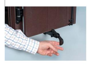
By lifting the stopping bow this is armed and the wall catch keeps open until the sash, when opening or closing, passes over it and unblocks it thus restoring the original position.
